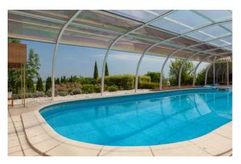
The high-strength profile system used in Aquacomet Endless Summer enclosures creates an opportunity to enclose wider pools. Fixed load bearing profiles are installed every 2 metres, while transparent, solid polycarbonate glazed doors between the profiles easily slide up to provide access to the pool. In this way the enclosure can be opened up to a height of 2.1 m along both sides. The segments are split horizontally into two parts and these
